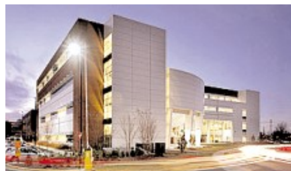
GENERAL CLASSROOM BUILDING
